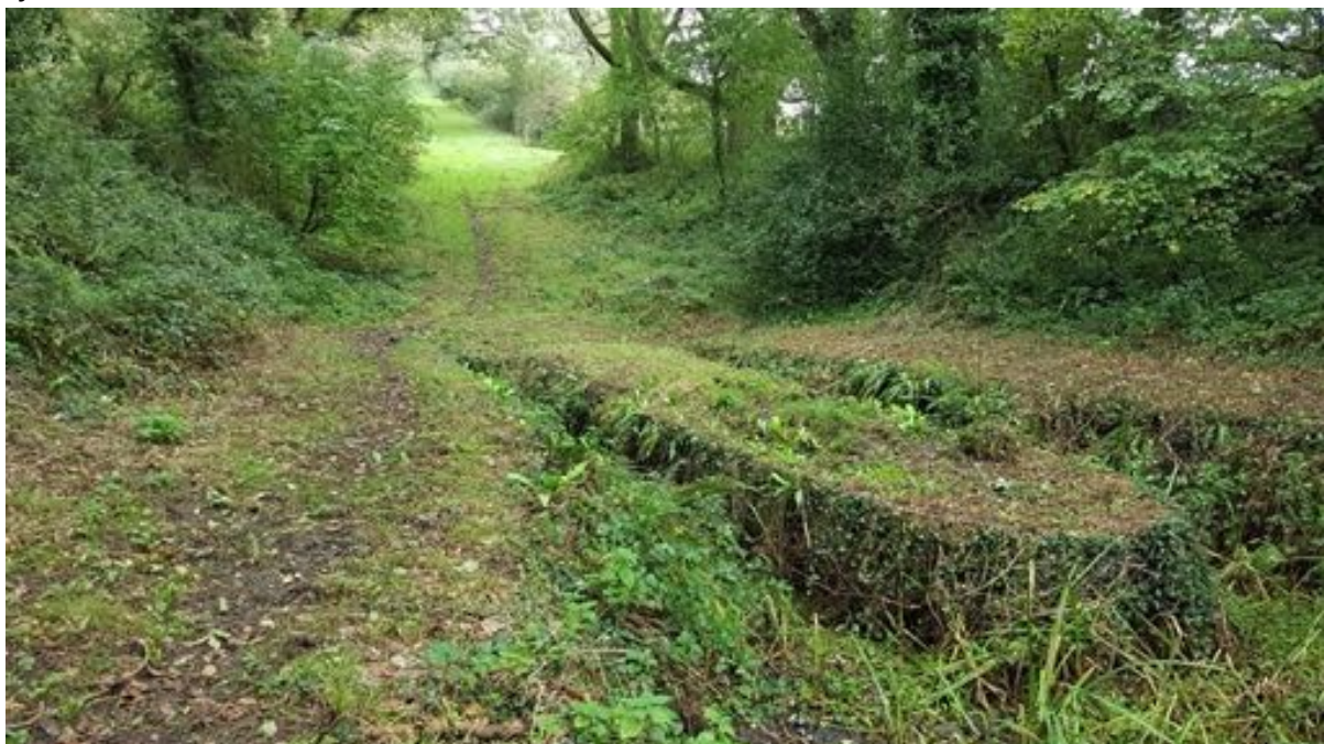
Below: Looking up the Hobbacott Incline Plane – used to haul wheeled tub boats to the higher section of canal.
